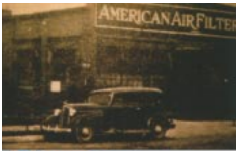
The original American Air Filter Company.
